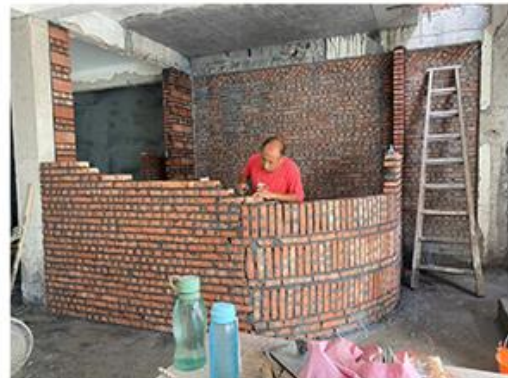
Figure 12 Building a wall and connecting a column
